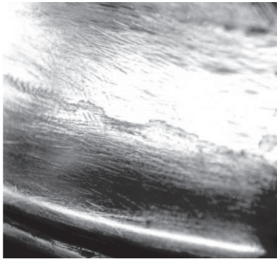
Figure 11. Amplified crack repair. The surface has been polished.
