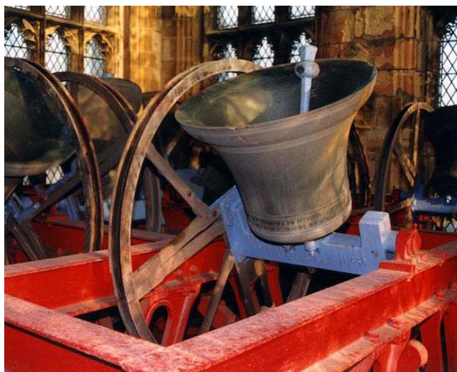
Figure 3-14 Bell being rung full circle
