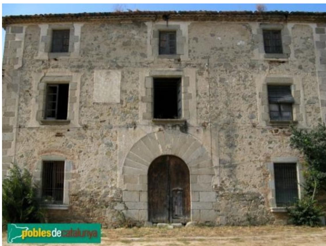
Argentona - Can Comalada (Foto: Albert Esteves, 2007)
